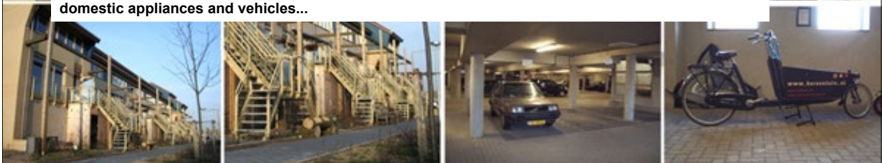
New logging in the Netherlands organised with common gardens, collective spaces, shared domestic appliances and vehicles...
